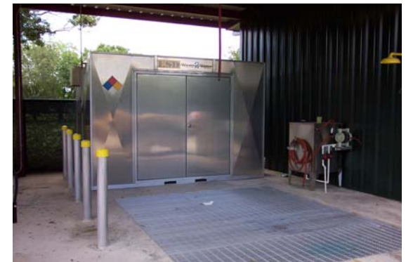
Chemical Handling Area
